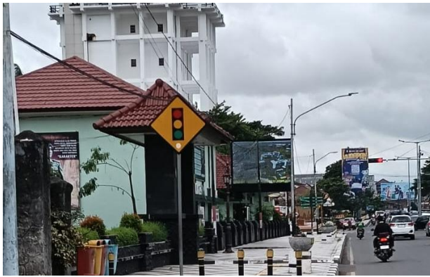
Gambar 11. Pedestrian Area Kantor TNI/CMP
